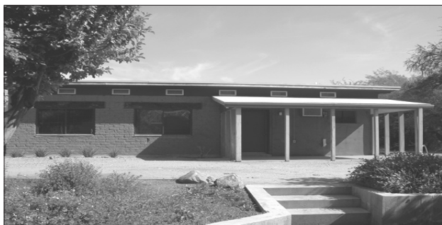
The above adobe structure, the first house in Water Village to be up and operating, is designed for point-of-use testing.
