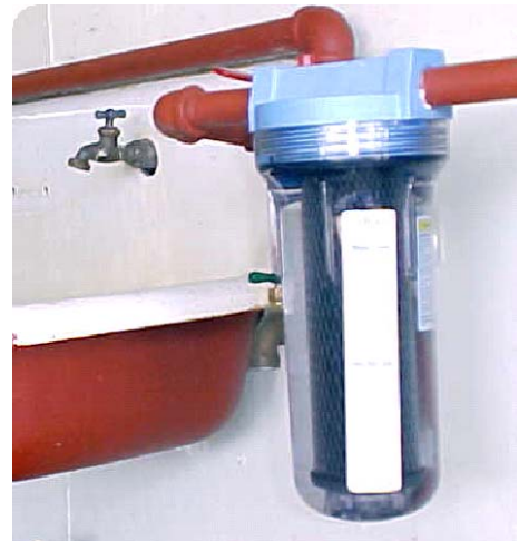
Carbon filters help your water taste better but they do not remove bacteria from the water.
