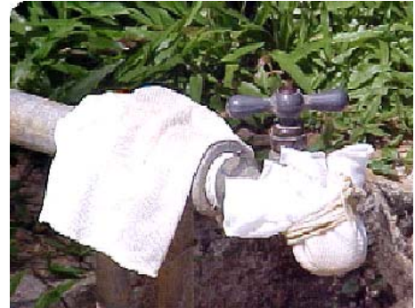
Dangerous bacteria can live in fabric filters. Use a wire mesh screen instead.
