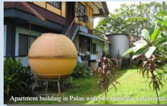
Apartment building in Palau with two rainwater catchments.
