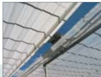
The retractable panels are operated by motors mounted on the roof. The thick panel on the left provides 50 percent shade; the thinner one on the right, 35 percent shade.
