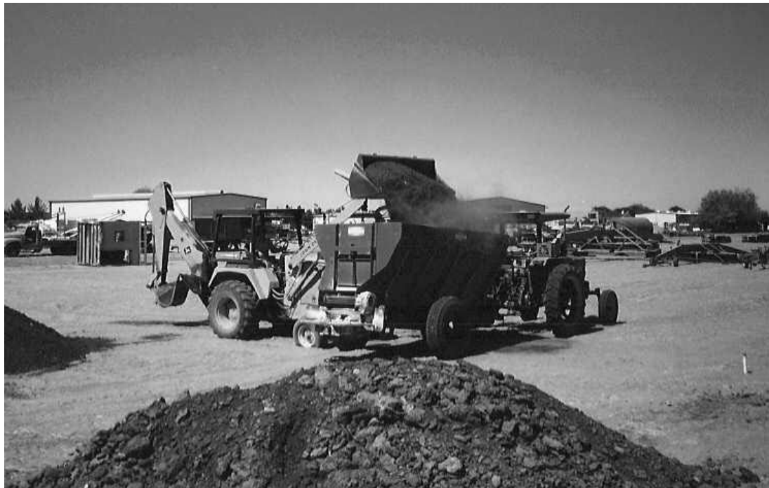
Figure 5. The spreader being loaded.
