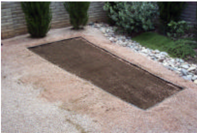
2. Remove 2—3 inches of soil and install border material.
