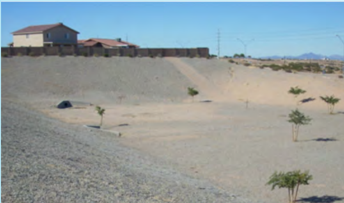
Figure 4. Stormwater Infiltration Basin in Yuma
