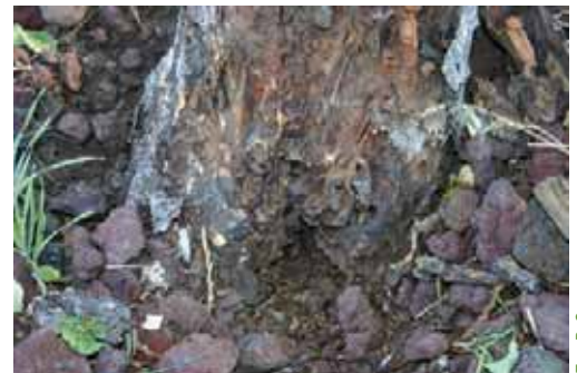
Photo 2. American hornet moth damage.
