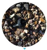
This drip emitter is connected to micro-tubing which is attached underground to a lateral line..
