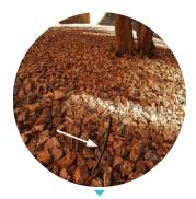
This micro-tube delivers water to the root zone of the tree. Under ground, it is attached to an emitter connected to a polyethylene tube.
