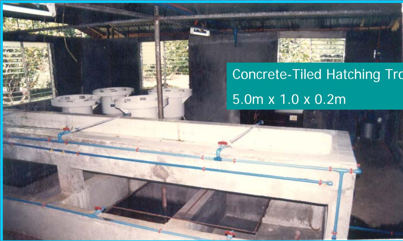
Concrete-Tiled Hatching Trough,
