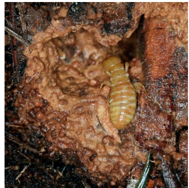
Dampwood termite gallery with high moisture. Note fecal pellets dissolving to form a muddy paste. Photo: Lynette Schimming
