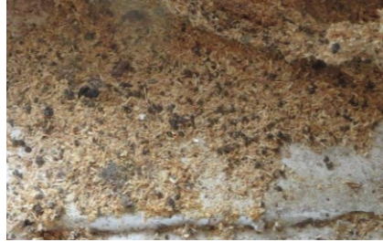
Carpenter ant damage produces piles of wood shavings (left)-Photo: Edward H. Holsten; Closer view of wood shavings mixed with ant body parts and other debris (right) - Photo: NY State IPM, Cornell
