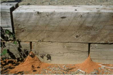
Carpenter ant damage produces piles of wood shavings (left)-Photo: Edward H. Holsten; Closer view of wood shavings mixed with ant body parts and other debris (right) - Photo: NY State IPM, Cornell
