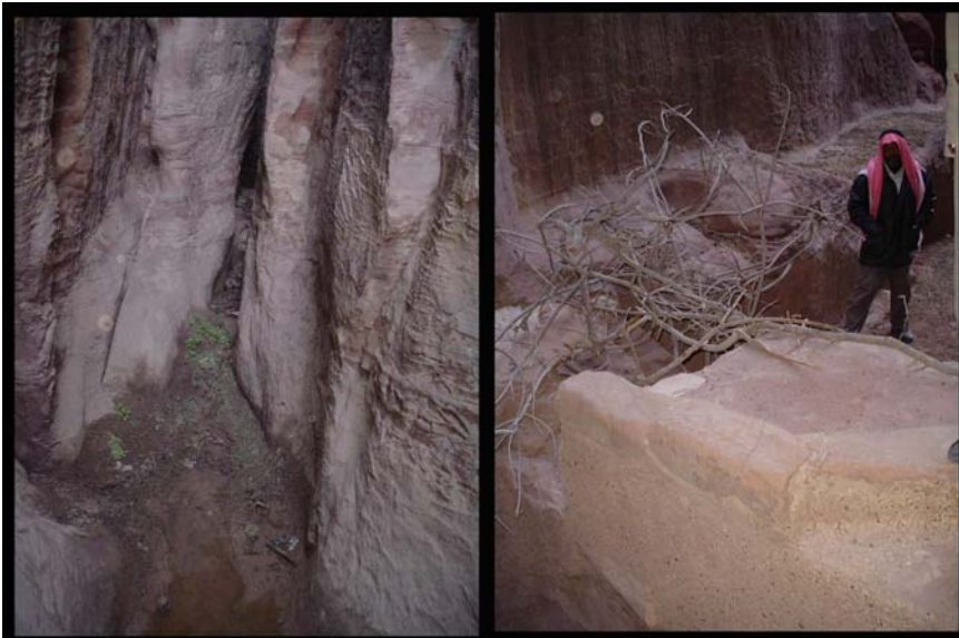
Figure 6a: Dam on Sidd al-Ahmar; silted, but in use
