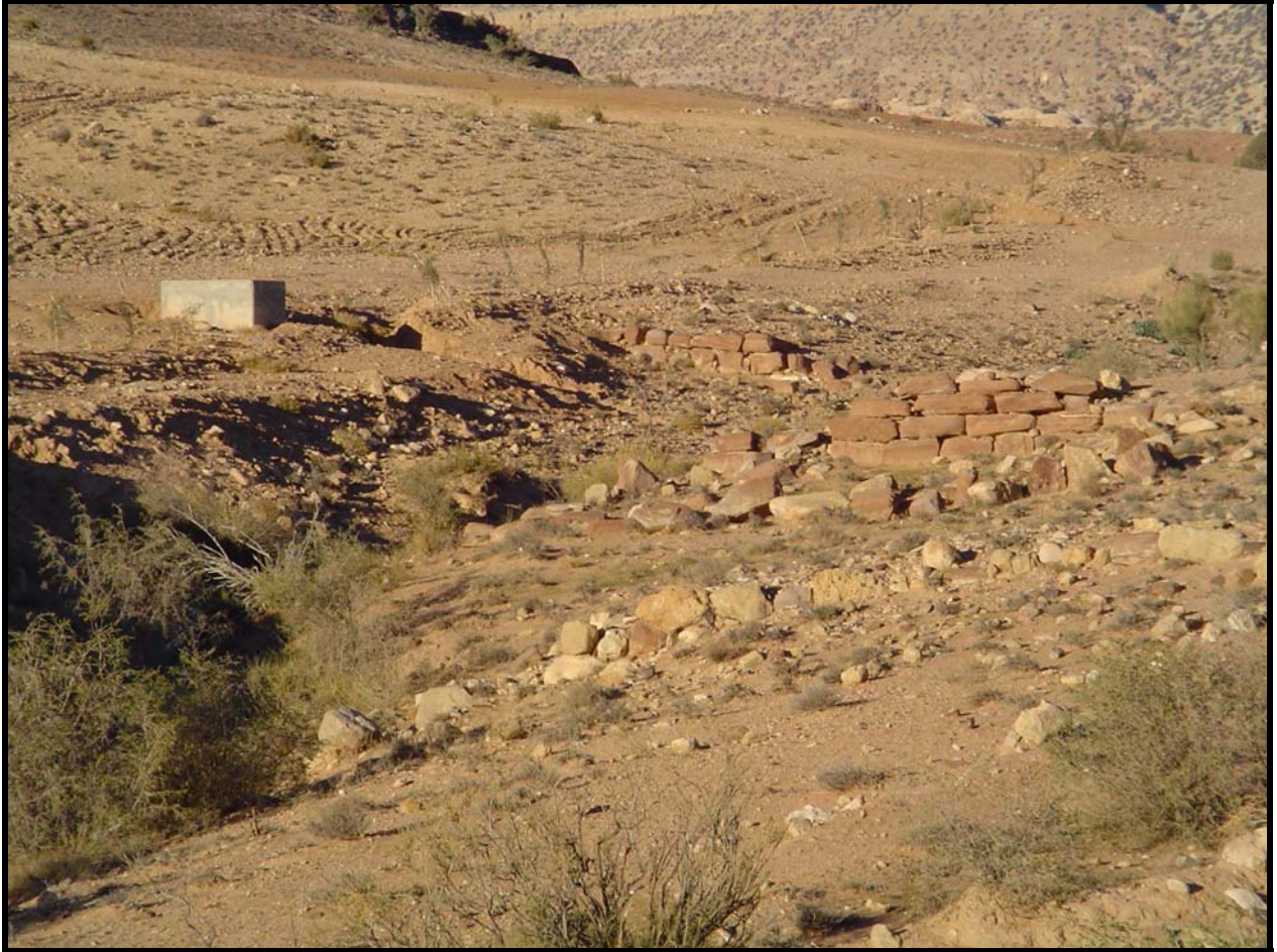
Figure 5: small dam on Wadi Umm al-Heiran -- period undetermined
